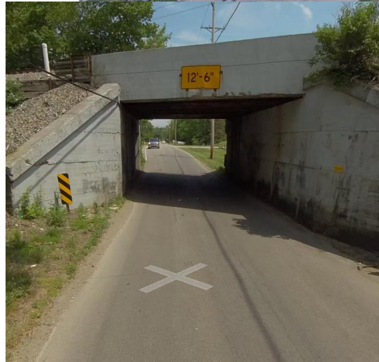
Franklin Trenton Road Underpass
