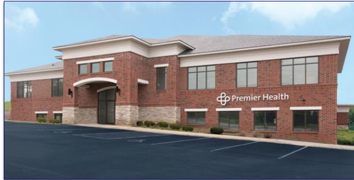
Middletown Cardiology Associates (Planned Unit Development)
